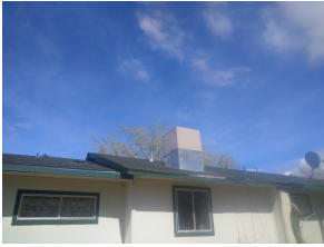
roof evaporative cooler
